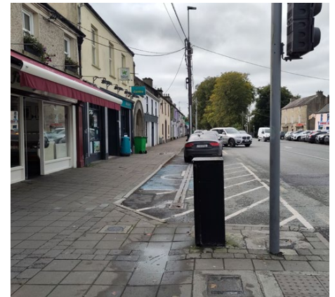
Clutter within the streetscape along Main Street, demonstrating the visual impact of overhead lines. Drainage is located within retrofitted accessible parking bays. Footpath materials are inconsistent across the town.
