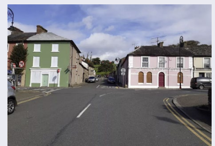
Refurbished residential accommodation in Cappoquin
