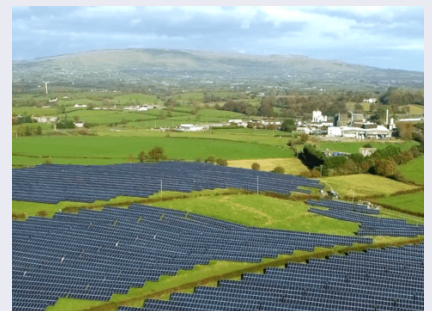
Dale Farm, example of Community Solar Farm
