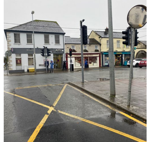
Narrow pedestrian crossing along Main Street
